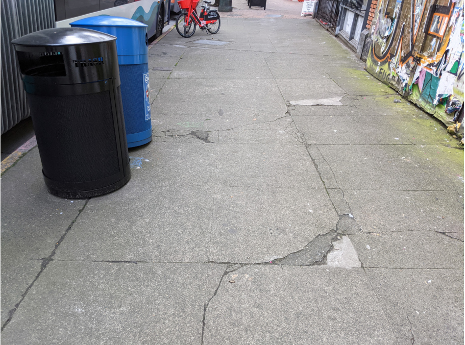
Looking south, in front of Busy Bee. Proposed extent of replaced concrete is the diagonal joint in front of the bicycle.
