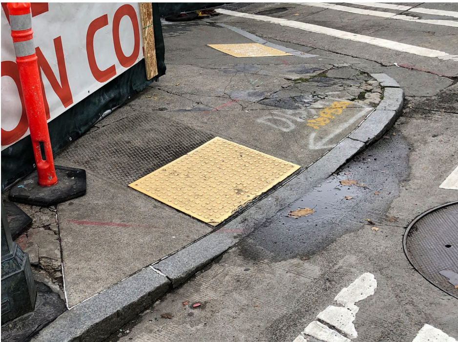
Granite curbs at corner with a small portion of concrete replacement curb where Yesler meets the corner.
