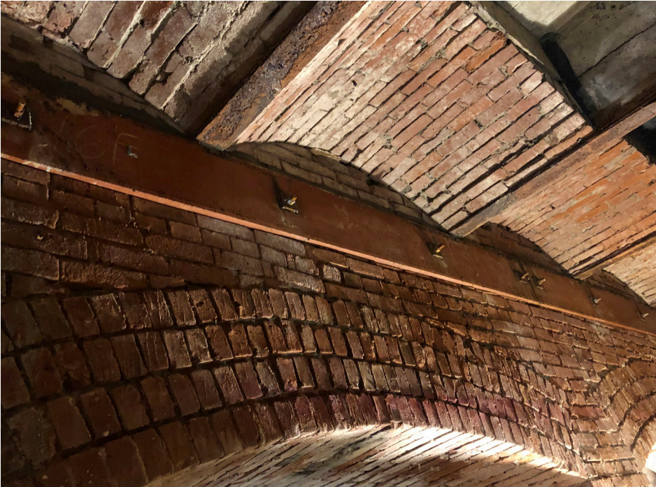
View of existing vaulted brick ceiling.
