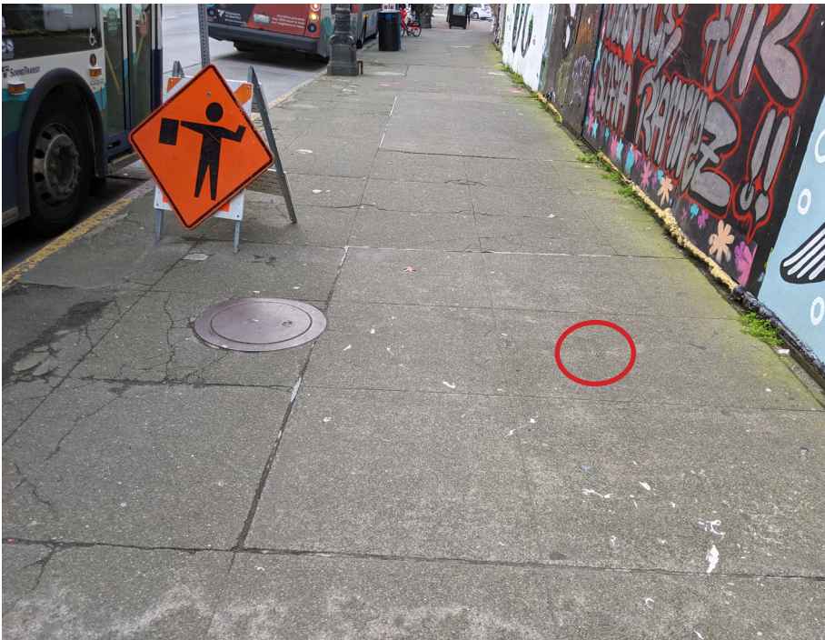
Looking south near the main entrance of Metropole. Hans Pederson stamp circled in red. The stamp is located in a panel that infilled an original glass prism location.
