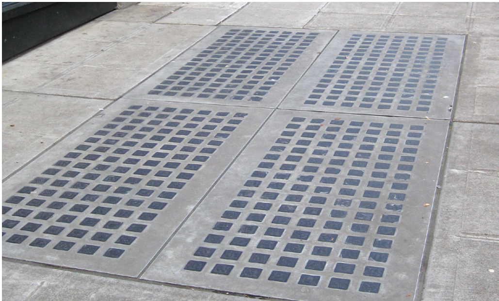
GLASS PRISMS PER THE PIONEER SQUARE PRISM GLASS DESIGN MANUAL
